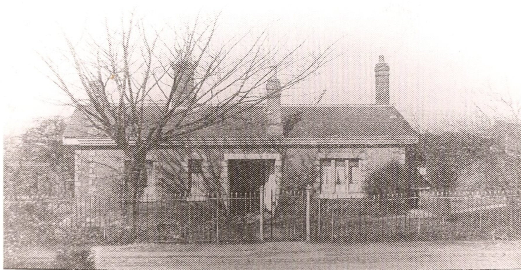
© Phil Jarvis - RHHG OLD RAILWAY STATION, CHIVE ROAD, REDDITCH.
